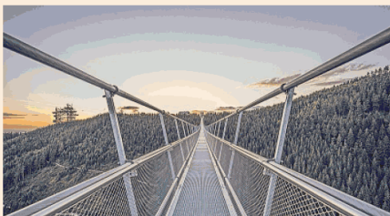
The new Sky Bridge 721, the world's longest suspension footbridge
