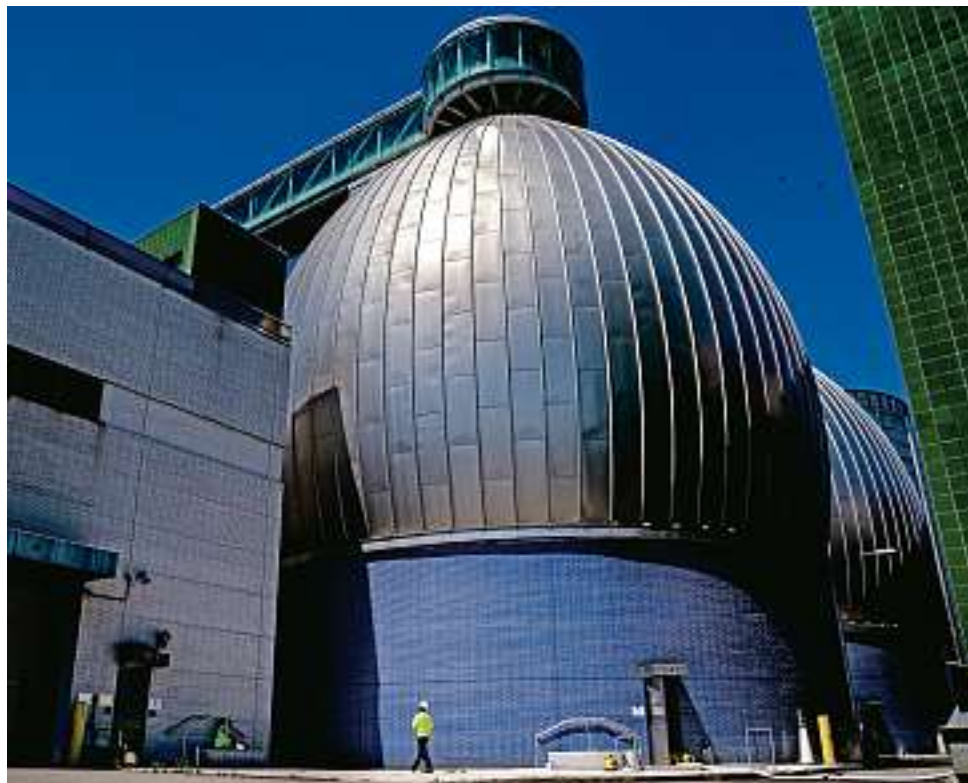
Health officials encourage vaccination. Above, Brooklyn's Newtown Creek Wastewater Treatment Plant
