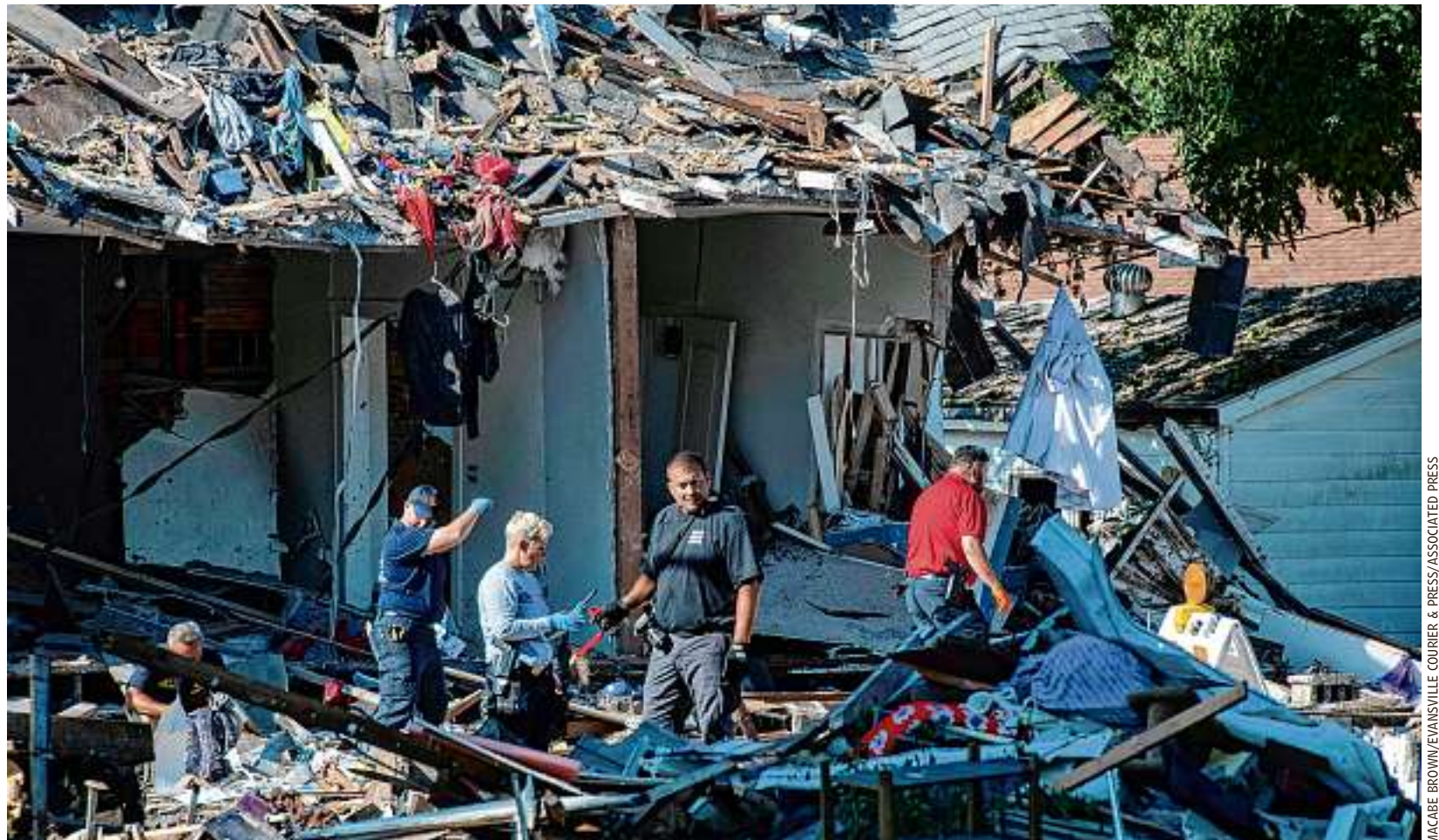
DISASTER: Officials Thursday were at the scene of a blast that killed three and damaged many homes Wednesday in Evansville. A gas line was being inspected, the fire chief said.
