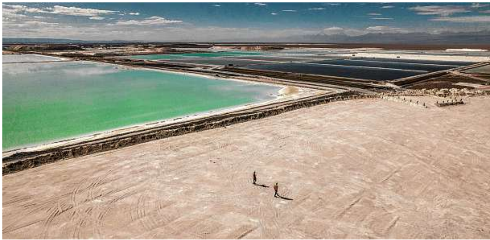
Evaporation ponds at an Albemarle Corp. lithium mine in Chile, above, are part of a water-intensive process that also involves a brine reservoir, below.
