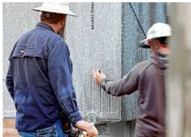
Workers inspected damage to a substation on Sunday.
