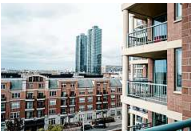
Tenants filed petitions with the city saying Portside Towers should be subject to rent control. The view from a tenant's balcony.
