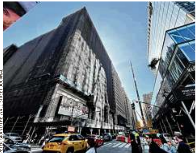
An office tower is planned for the site of the Hotel Pennsylvania.
