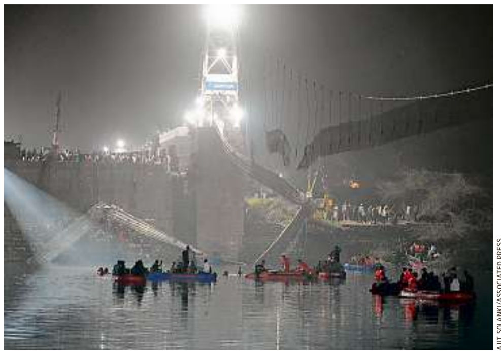
Rescuers on Monday search the Machchhu River for survivors after the collapse of bridge.
