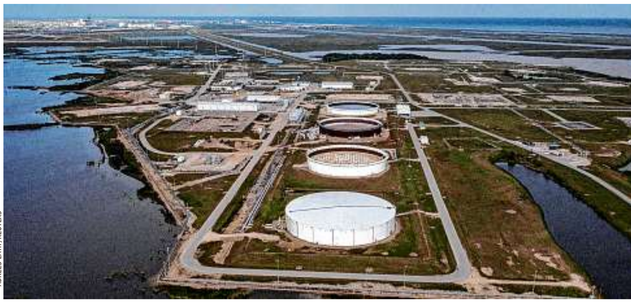
The Bryan Mound Strategic Petroleum Reserve, an oil-storage facility, in Freeport, Texas.
