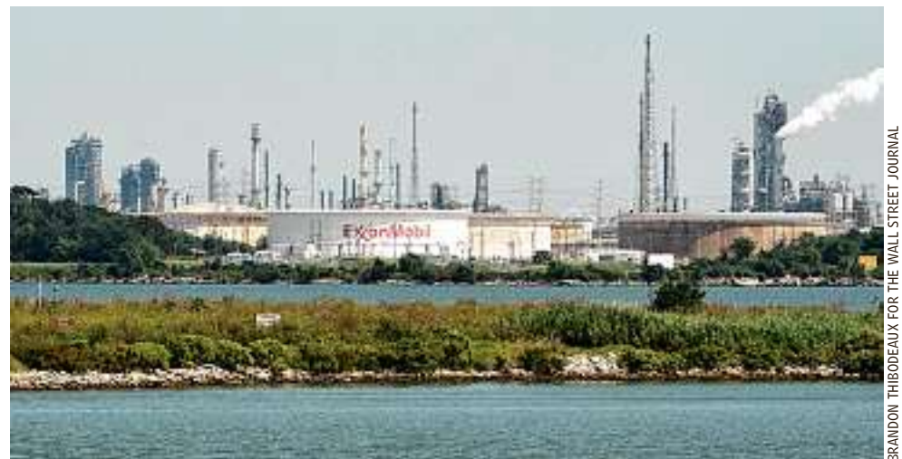
Exxon plans to offer carbon capture services to other companies. Its Baytown, Texas, facility.
